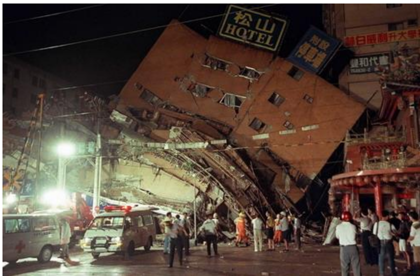
Collapsed building after 9 21 Jiji Earthquake
