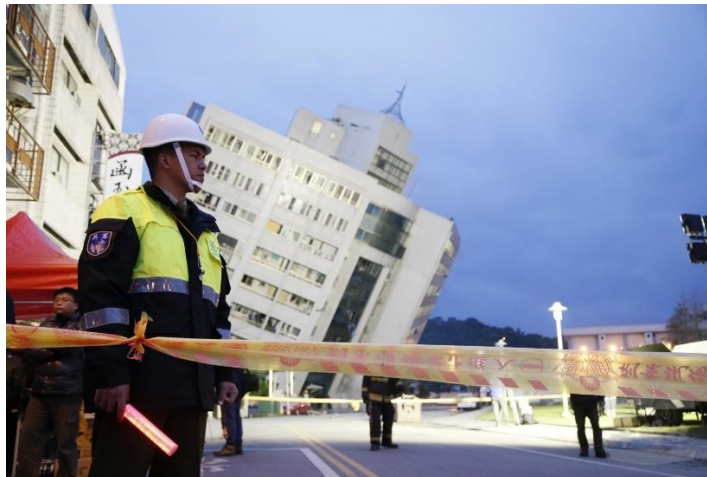
Yun Men Tsui Ti building in Hualien, After Feb. 6, 2018 Quake
